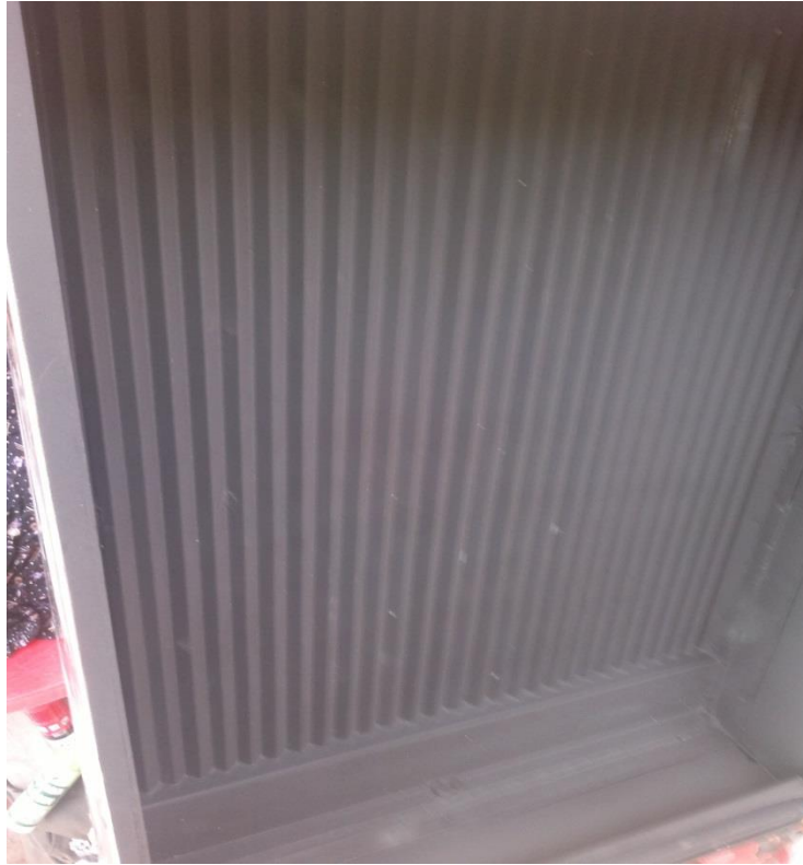
Appendix A7: After painting the collector
