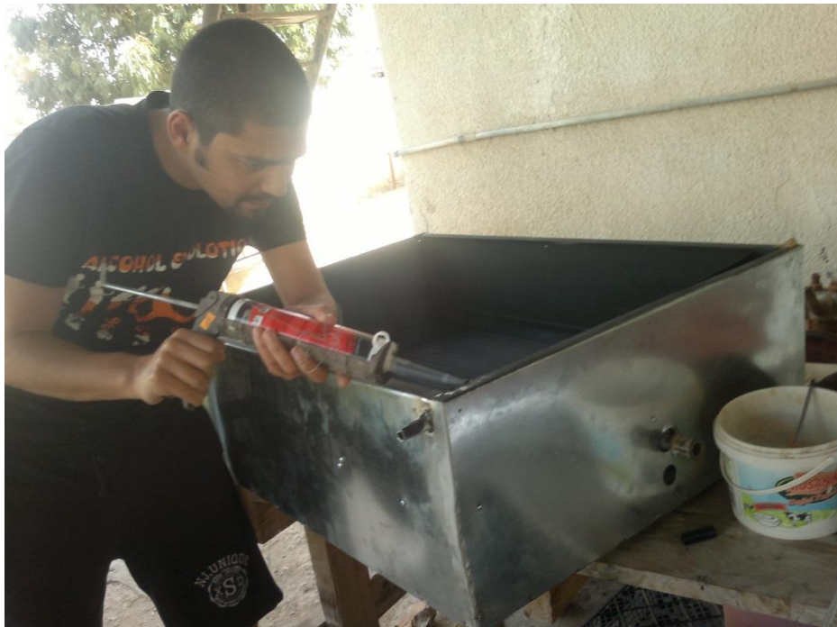
Appendix A8: Leakages are blocked with silicone
