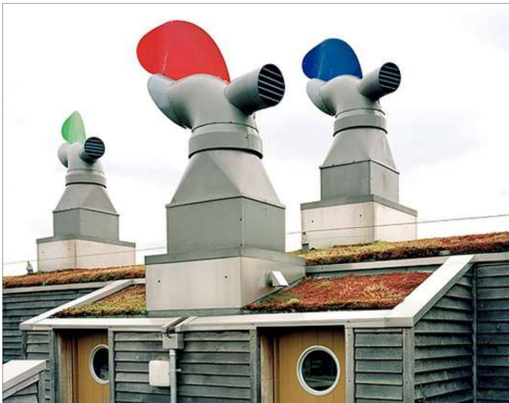
Figure 2.1: Wind scoop on top of the Beddington Zero building. (Skeele, 2011)
