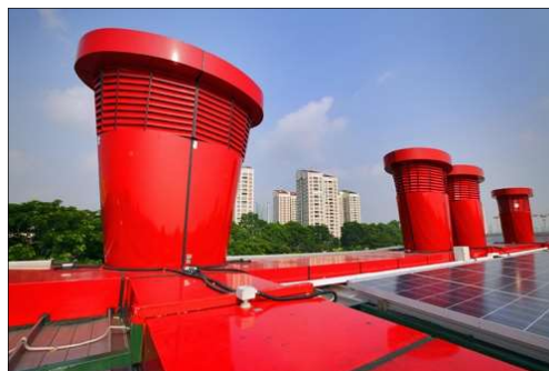
Figure 2.9: Chimneys on roof level. (Yudelson Associate, 2011)
