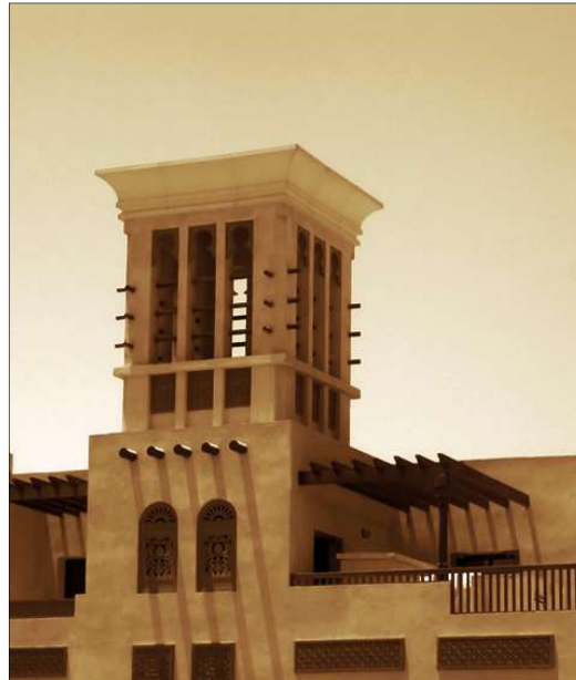
Figure 2.6: Wind catcher at roof level of the building. (Mahyari, 1997)
