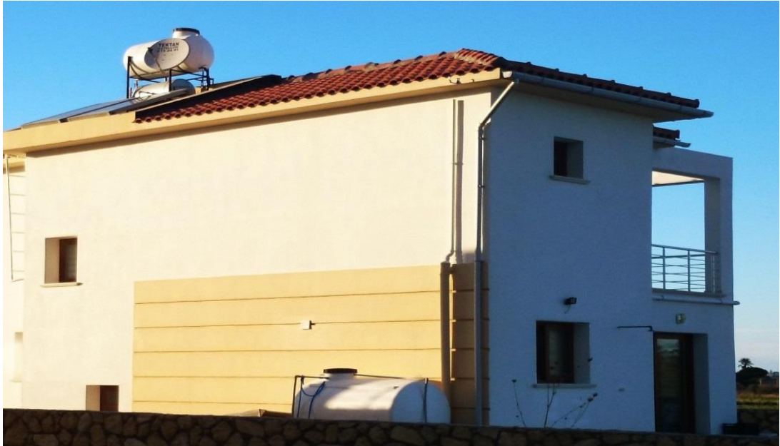
Figure 1.1. Photograph of a typical dwelling adapted with ground and roof tanks and an SWHS in North Cyprus.
