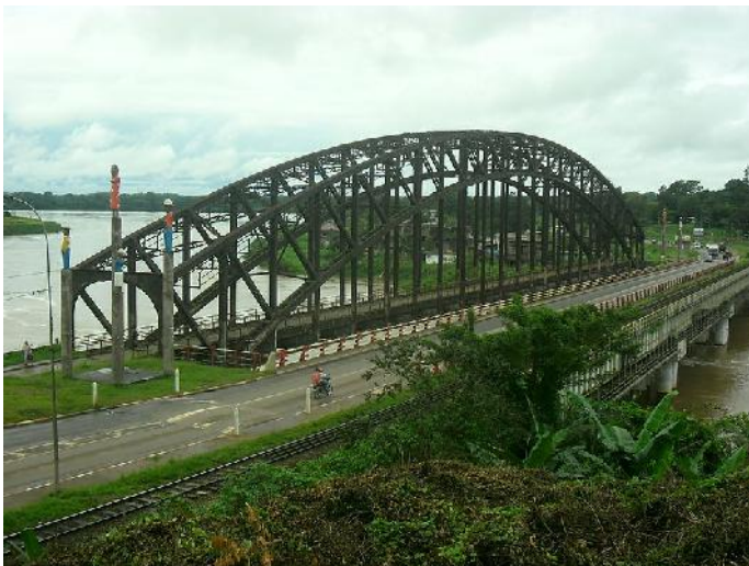
Figure 6: The Sanaga Bridge
