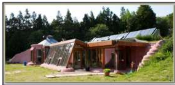
Figure 11: View of Earthship Brighton
