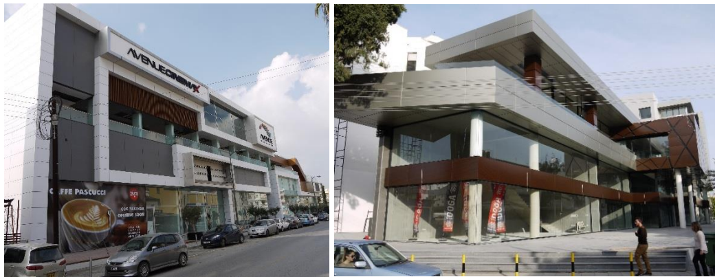
Figure 3.23: New construction in Mehmet Akif Street
