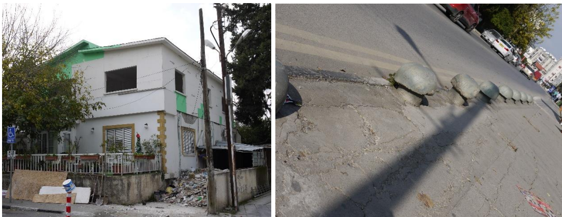
Figure 3.28: Maintenance of buildings and pavements in the Mehmet Akif street
