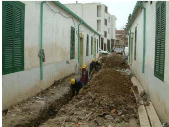
Figure 5: Samanbahce during restoration (16).
