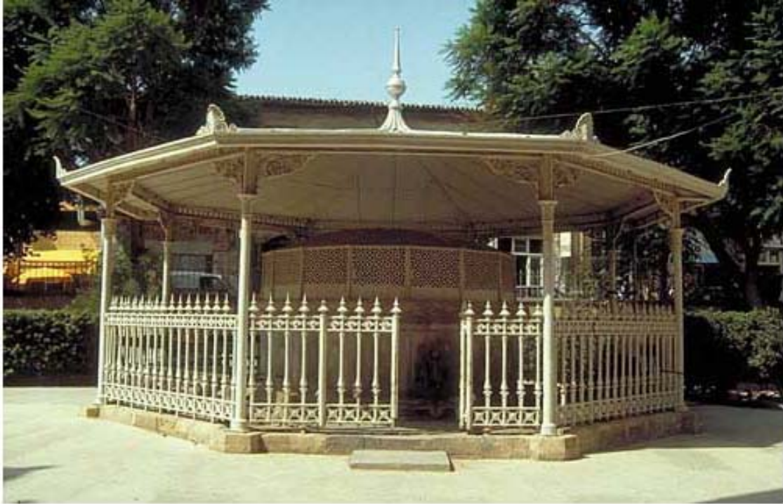
Figure 7: Fountain of the Selimiye Mosque, Nicosia
