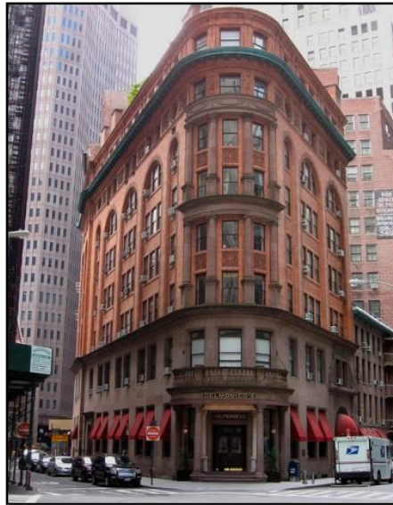
Figure 15: Arcades, balconies and bay-windows are the most significant parts of the corner buildings Delmonico's Building, New York City (URL 15)
