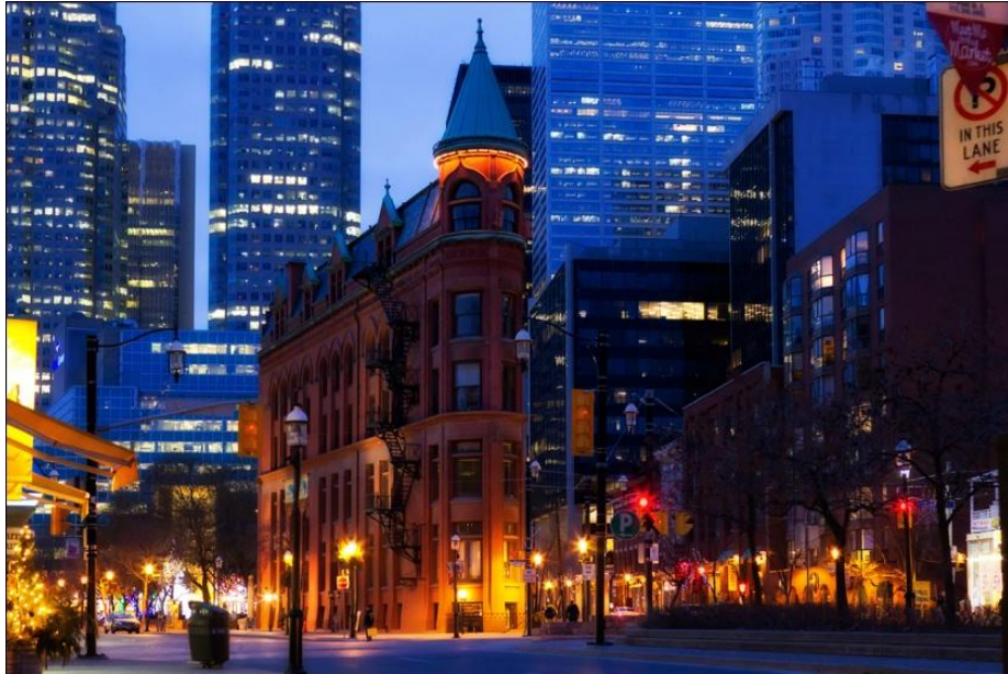
Figure 2: Corner building as a focal point. Gooderham Building (URL 2)
