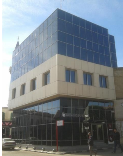
Figure 63 : Building 16 [Yakin Dogu Bank (Taken by Author)]
