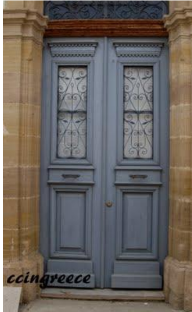
Figure 44: Fanlight above the door, wooden material, glass and iron (URL44)
