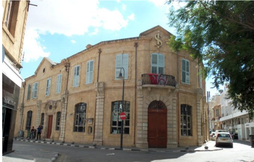
Figure 49 : Building 2. [Iş Bankasi] (Taken by Author)
