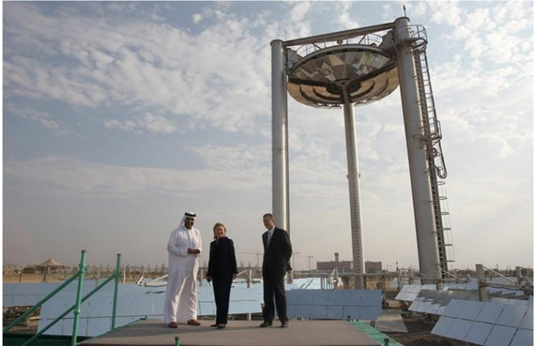
Figure 2.9: Centralized Solar PV System in Masdar City [URL 1]. This figure shows the innovation and advanced technology use in Masdar City.
