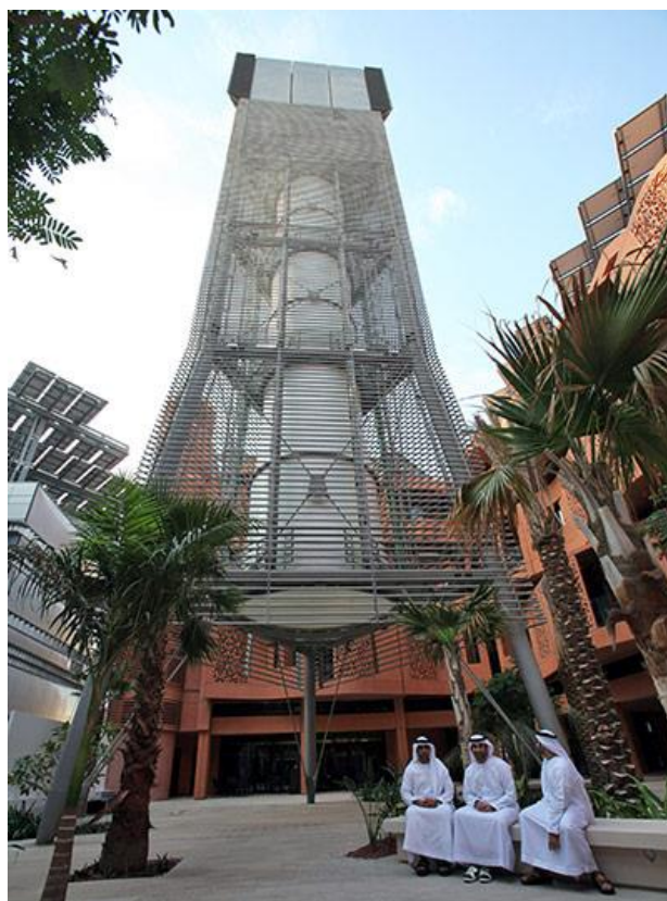
Figure 2.10: The Teflon-Coated Wind Tower in Masdar City [URL 1]. This efficient technology in Masdar City is used to provide cooler streets in city than surrounding desert.
