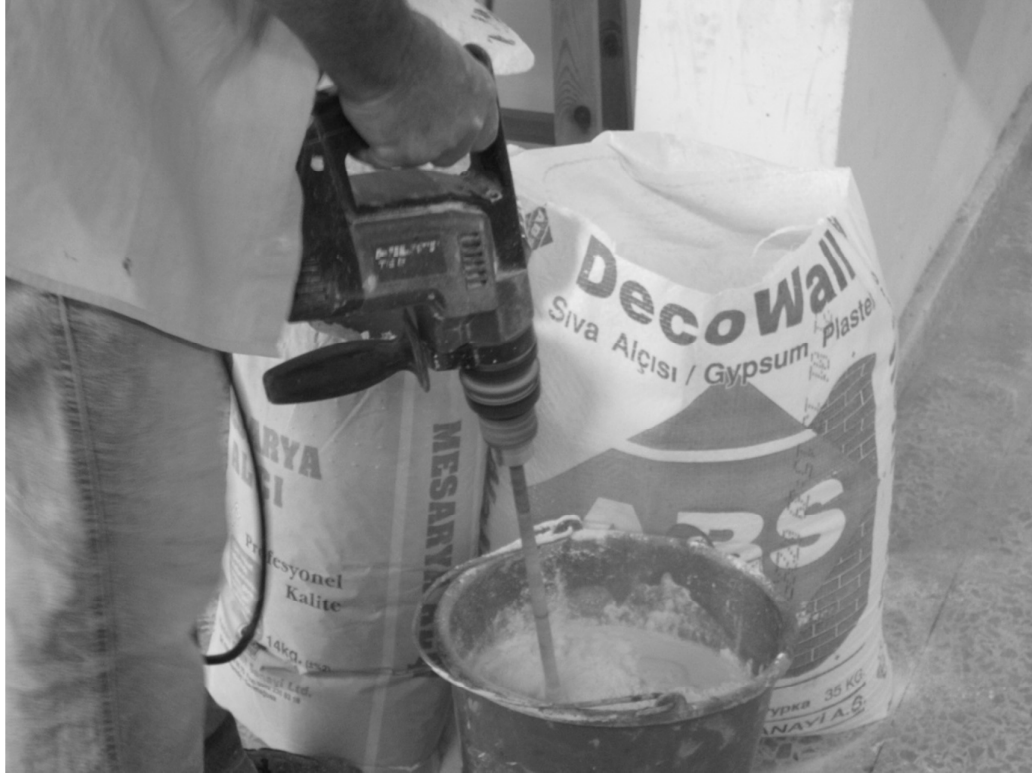
Figure 3.20: Preparing Gypsum Plaster with ABS Deco-Wall and Water
