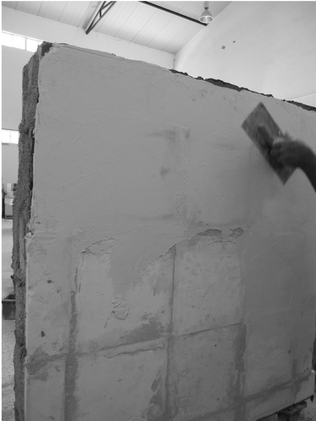
Figure 3.23: 1mm Thick of ABS Gypsum Plaster was Applied on the Surface of LCMP Samples
