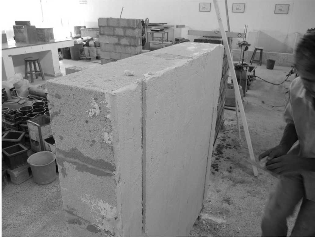
Figure 3.21: 10 mm of Gypsum Plaster Applied on the Wall Specimen
