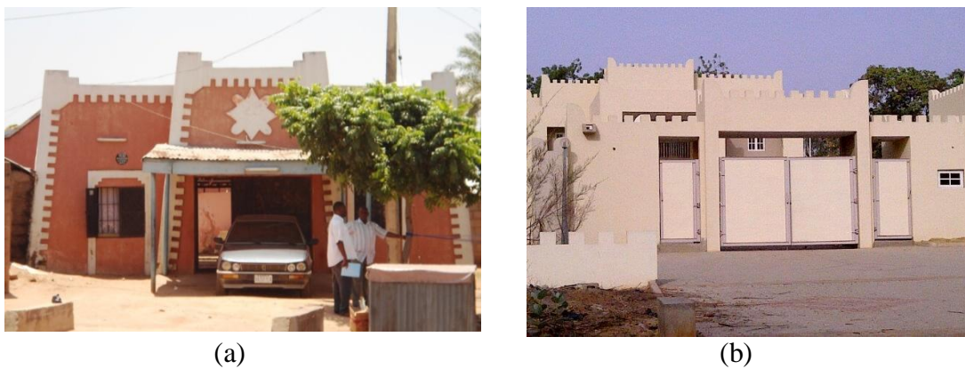
Figure 4.12: Pictorial views of postmodern buildings showing colors and textures. (Photo by author)
