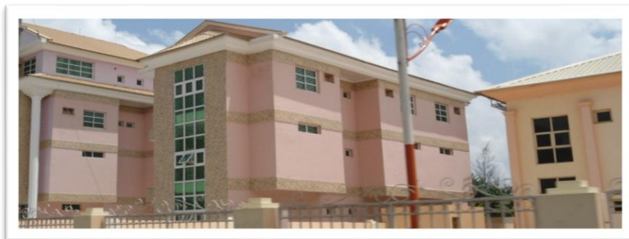
Figure 3.10: Shows postmodern commercial building in Kaduna with effects post-colonial effects, (photo by author)
