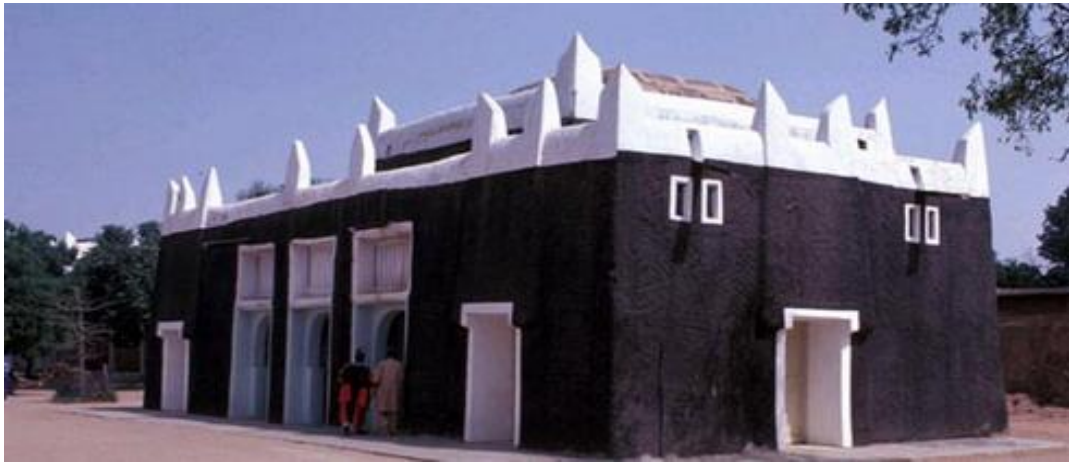
Figure 3.16: Shows traditional residential (museum) with pinnacle (zanko) and rawani. (Photo by Author)
