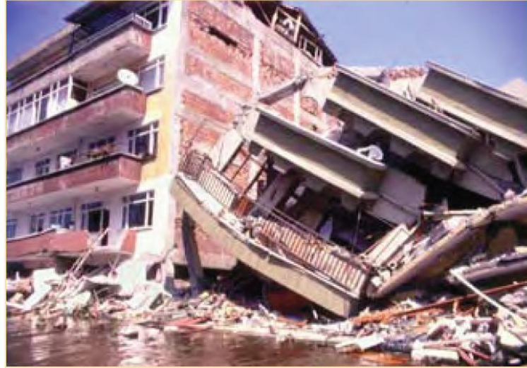
Figure 3.25. Illustration of the Destruction Triggered by Weak Column-Strong Beam Structure (Gulkan et al. 2002)
