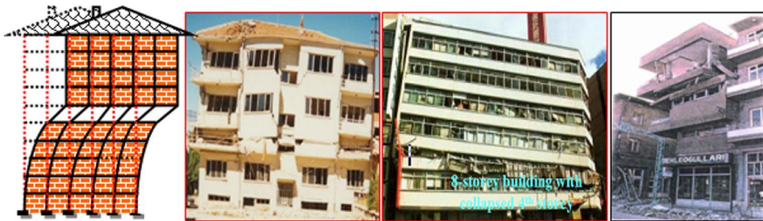
Figure 3.16. Failure of Middle Floors under Earthquake Loads (Doğan 1986)
