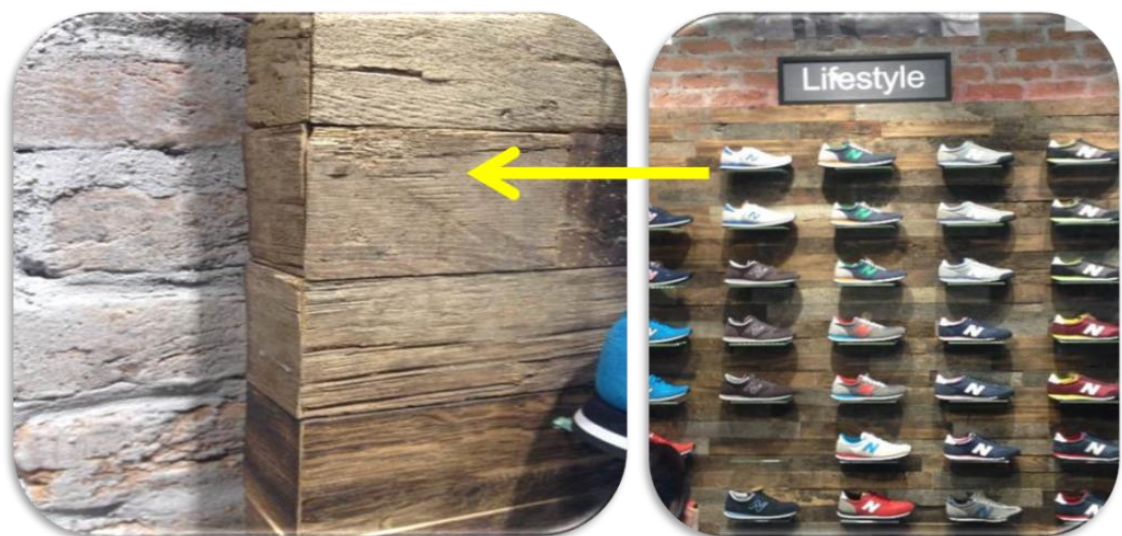
Figure 87: Using recycled timbers to create texture- Istinye Park interior design
