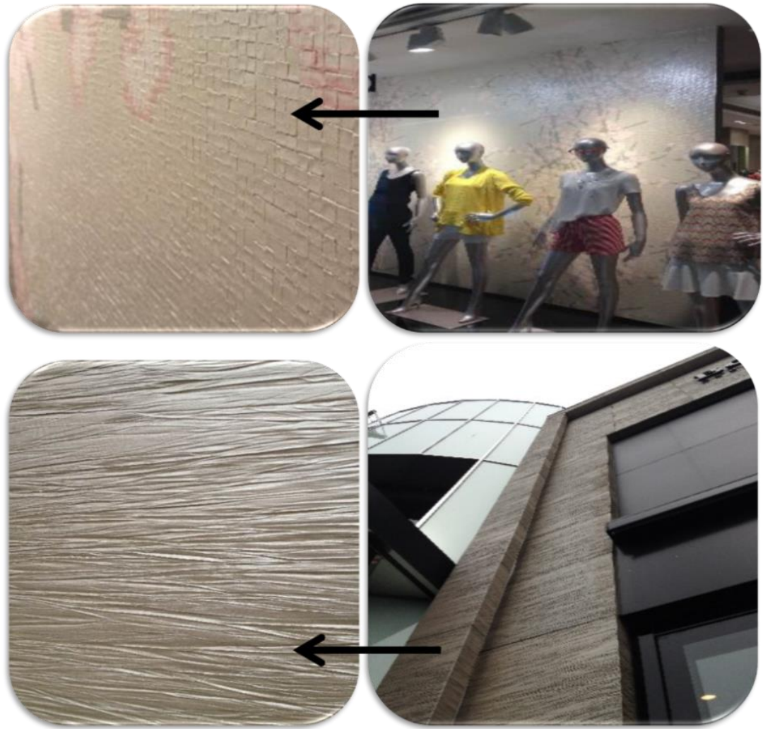
Figure 90: Using liquid materials on original surface and scratch them to create texture in interior design of Istinye Park
