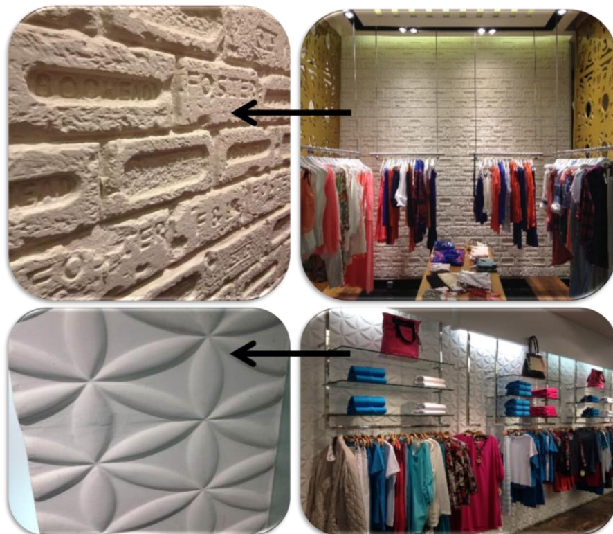
Figure 92: Molding liquid materials to create texture in interior design of Istinye Park
