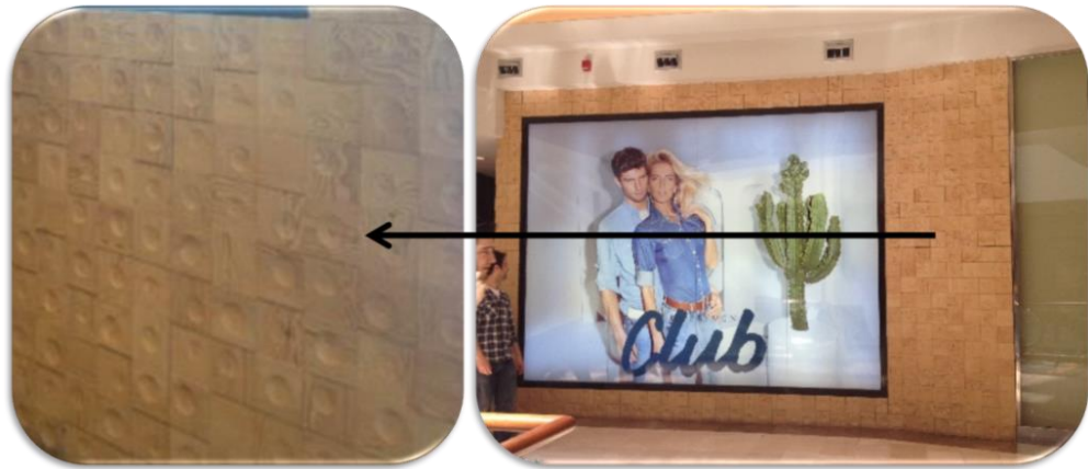
Figure 91: Using solid materials and scratching them to create texture in interior design of Istinye Park
