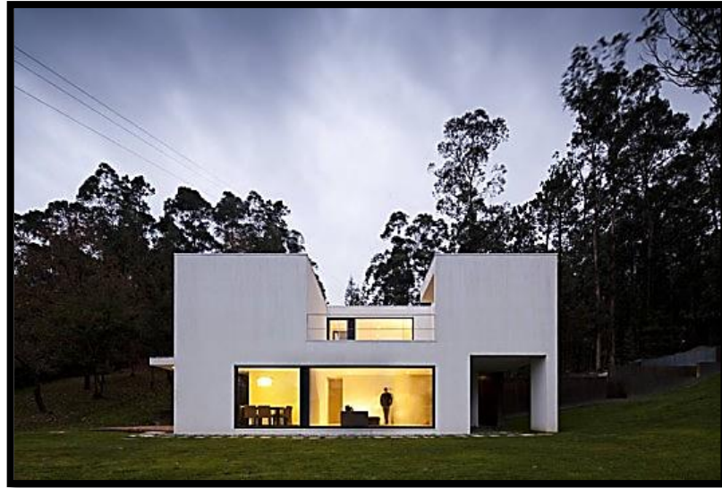
Figure 17. Private House in Barcelos (Garrido, 2012)
