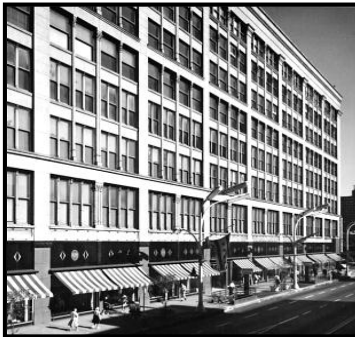
Figure 16. Reinforced Concrete Frame Structure (Urbanosis, 2007)
