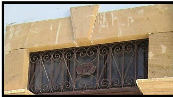
Figure 67. Fan Light Window of I. British Period-1913
