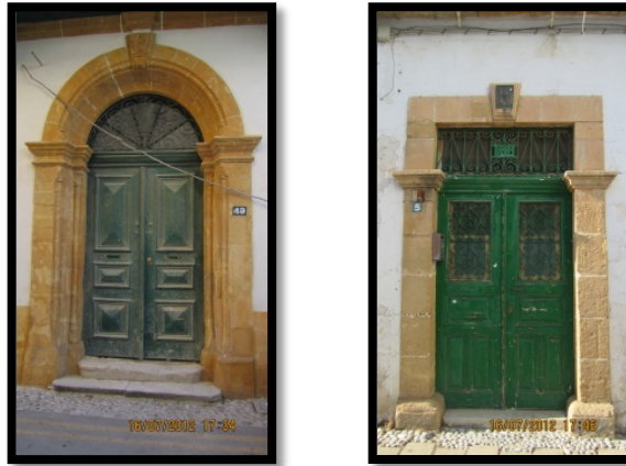
Figure 36. Doors with Semi-Circular and Rectangular Fanlight Windows
