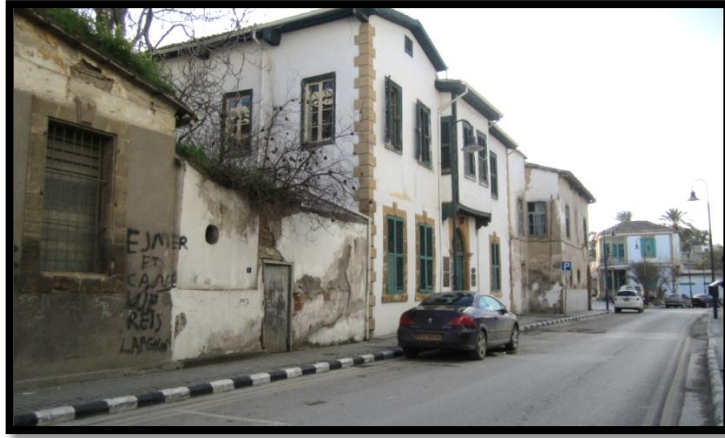
Figure 47. View of Vacant and Renewed Building's Façade
