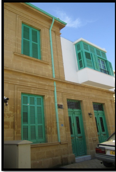
Figure 34. Yellow Stone Building of Second British Period-1934
