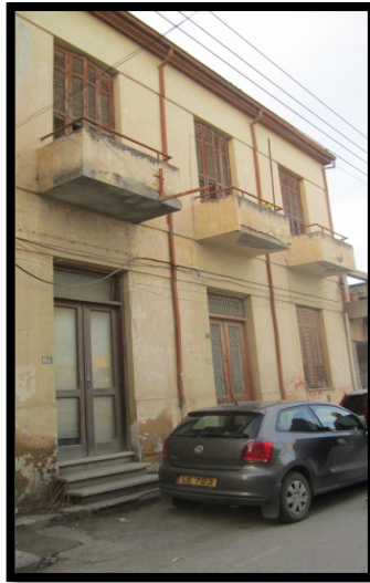
Figure 32. Reinforced Concrete Structural System- 1948
