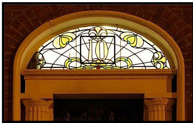
Figure 20. Fanlight and Number of the House (Bridge, 2009)
