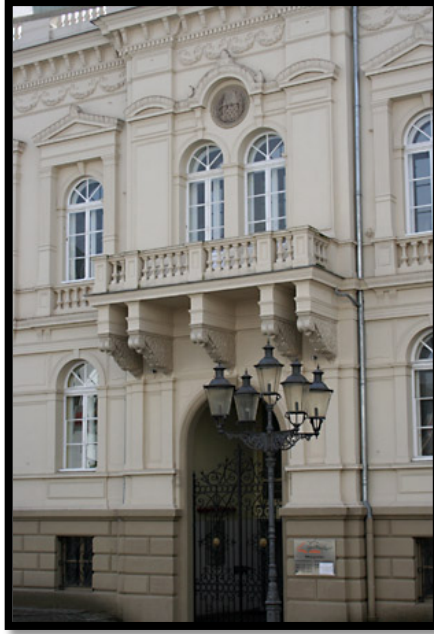
Figure 21. Balcony on the Town Hall Building in Iserlohn (Mecomber, 2013)
