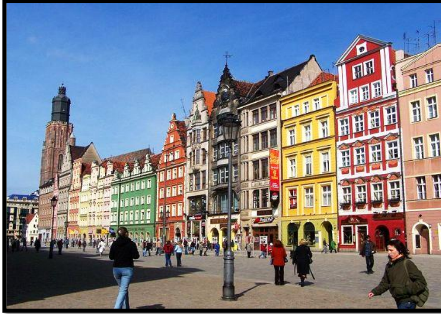
Figure 19. Colored Façade in Historic Town at Wrocław's Main Market Square (Mehlich, 2013)
