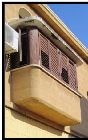
Figure 63. Last Bay Window of Building 34- 1948
