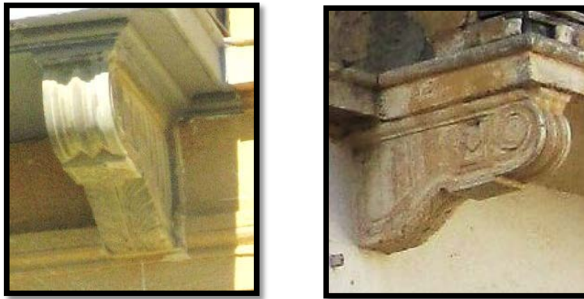
Figure 69. Stone Brackets in the Buildings 29, 33
