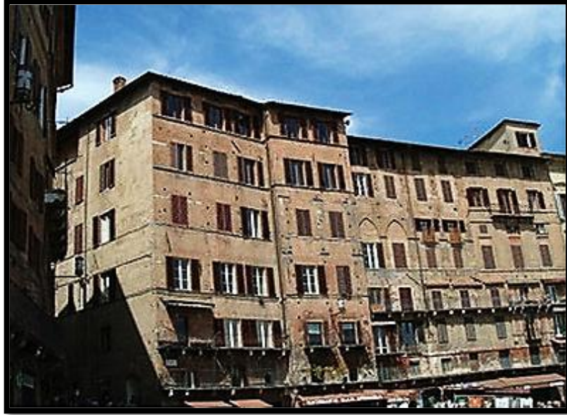
Figure 9. Low Share of Window Area at the Piazza Del Campo in Siena of Italia (Konstantinou, 2013)
