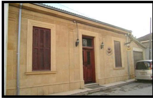
Figure 46. Use Yellow Stone as a Local Material
