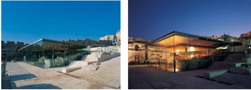
Figure 32: The building concentrates on using light-weight materials such as steel, wood and glass to reduce stress from the original building (Source: Xiaolu Li., 2010)
