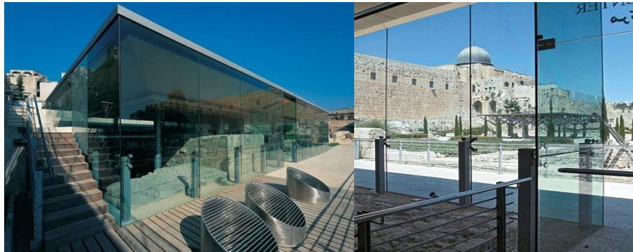
Figure 23: Selected glass prevents ultra-violate light from entering and damaging the artifacts (Source: Xiaolu Li., 2010)
