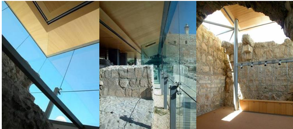
Figure 29: Light weight wooden and steel walls, combined with glass walls (Source: Kimmel, 2011)
