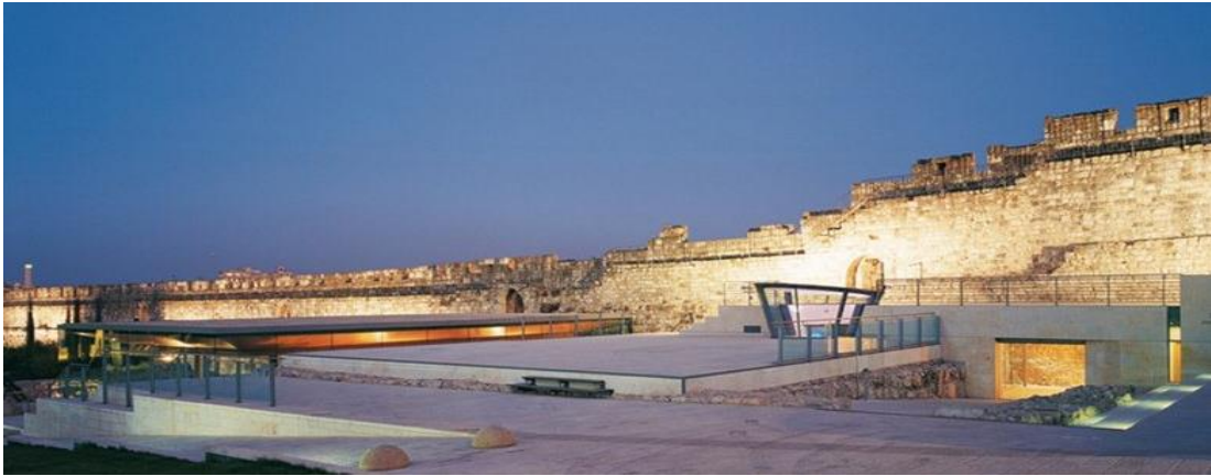
Figure 18: The roof being built as low as possible to be parallel with the palace floors (Source: Xiaolu Li., 2010)
