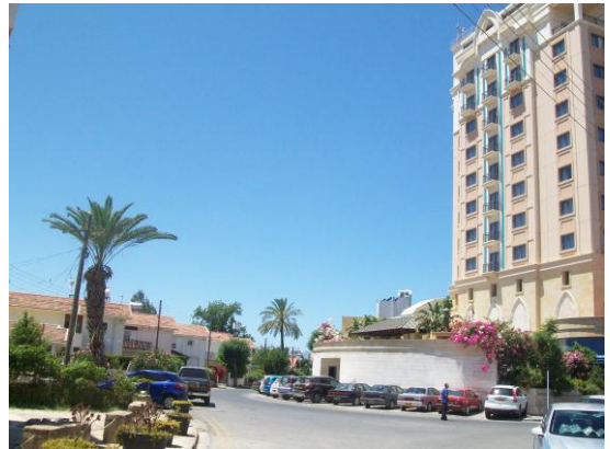
Figure 20: Disturbed the street skyline and overshadowing on row houses by Merit Hotel,
