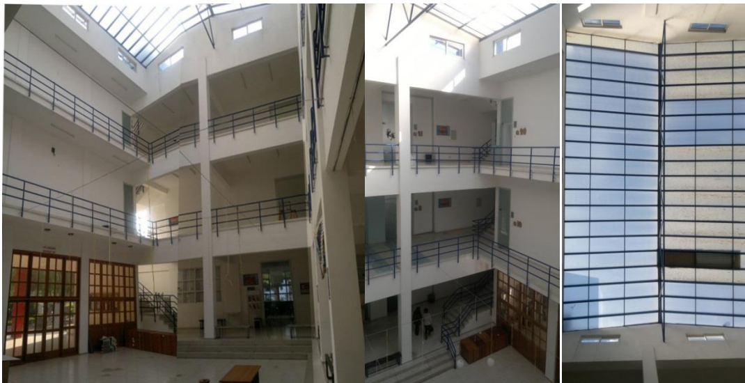
Figure 40: Interior Views of the Coloured Building's Atrium
