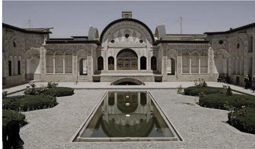
Figure 4: The Main Courtyard of Tabatabaei House, in Kashan, Iran
