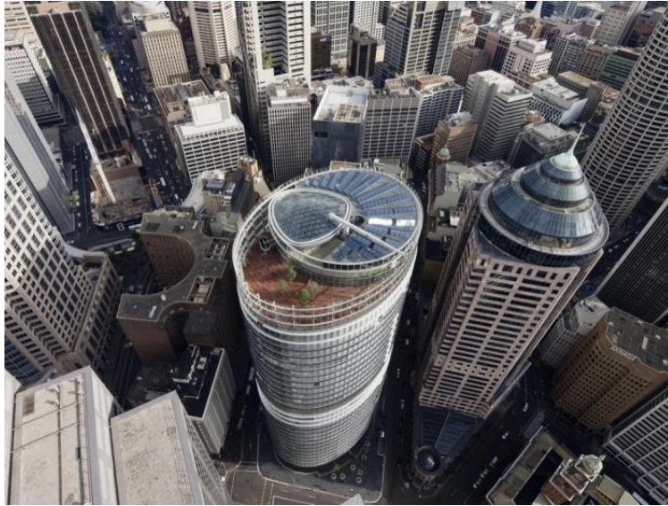
Figure 34: A General View of 1 Bligh Office Tower
