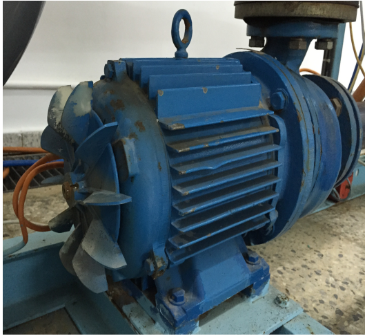
Figure 3.5: Cleaning the pump
