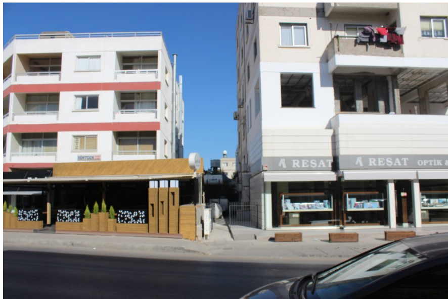
Figure 3.6. Lack of Continuity in Roofline
