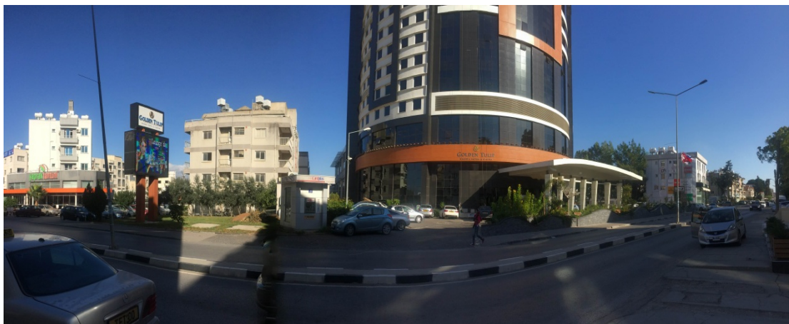
Figure 3.9. Discontinuity and Irregular Rooflines and Separated Building Blocks
