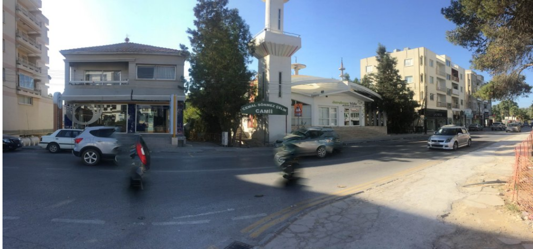
Figure 3.11. Discontinuity and irregular rooflines and separated building blocks
