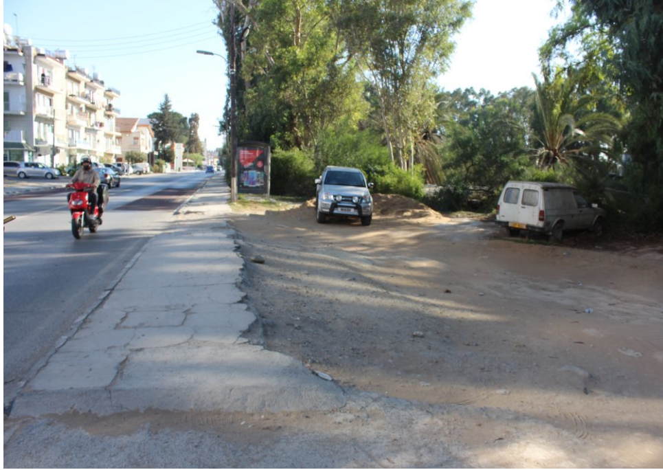
Figure 3.14. Poorly Maintained Pathways along the Sidewalks
