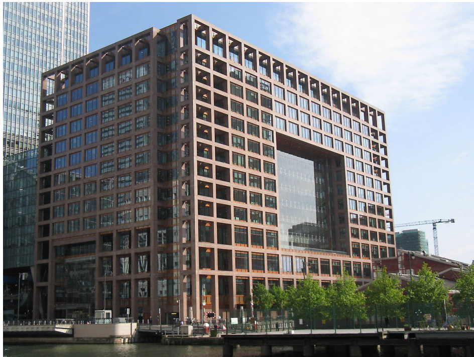
Figure 2.8. Façade, Office Building, London, United Kingdom (URL27)
