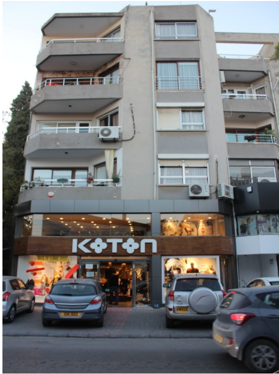
Figure 3.8. Residential Building in Mix with Shops
