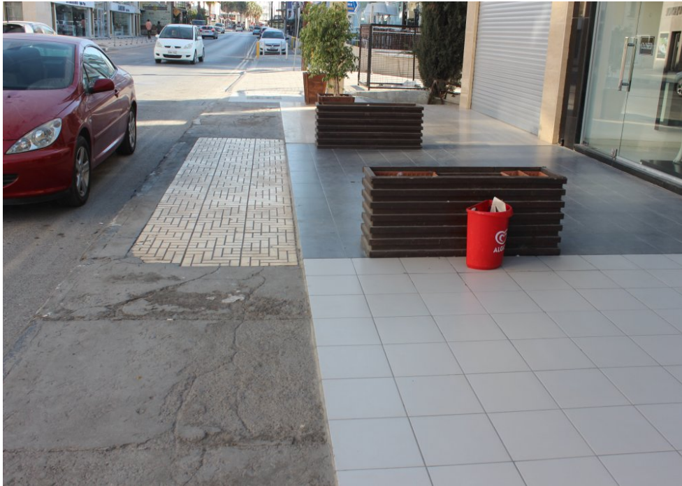
Figure 3.16. Flooring of Sidewalk with Different Material, Shape and Heights
