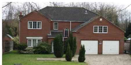
Figure 2.17. Detached Houses/Single-Family House
