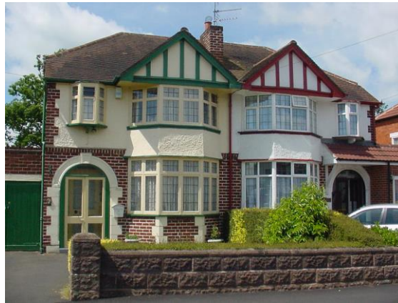
Figure 2.18. Semi Detached House
