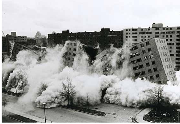
Figure 4: Demolition of Pruitt-Igoe Housing Development designed by St. Louis Architects in 1951, demolished at July 15th 1972, (URL 1)
