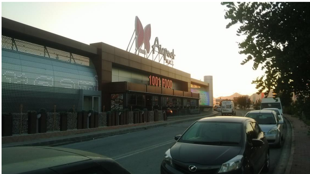
Figure 61: Covering of Building with Curved Perforated Steel Sheet
