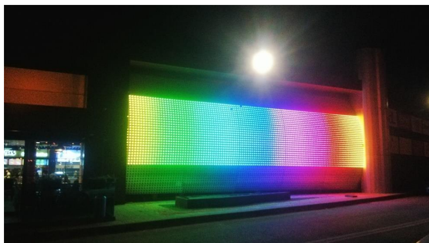
Figure 60: LED integrated façade of 1001 Airport Mall
