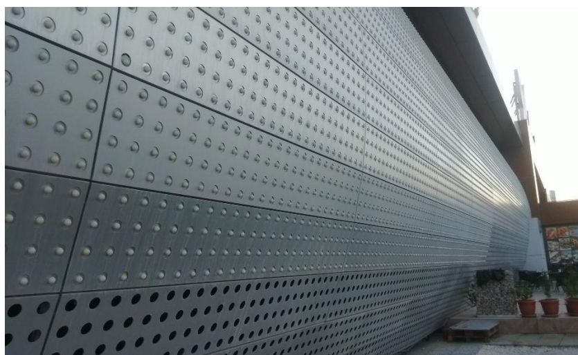
Figure 68: Integration LED to Fake Façade of Curved Steel Sheets
