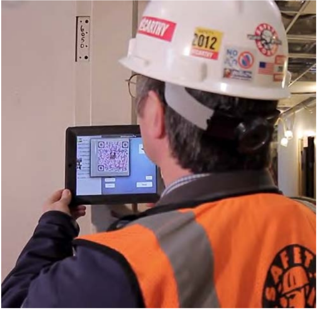
Figure 16: Superintendent using BIM Anywhere to scan QR codes for quality control
