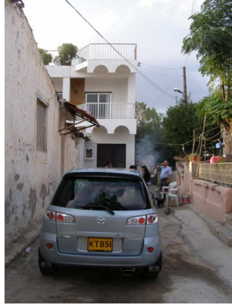
Figure 39: View of ST4 before the renovation
