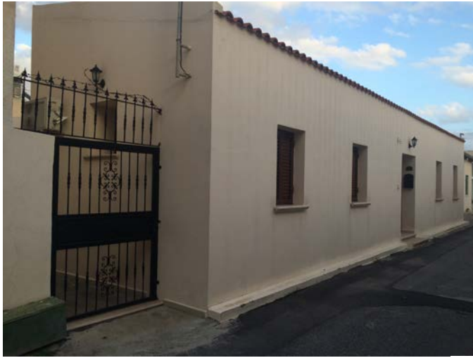
Figure 48: One Storey building in ST7
