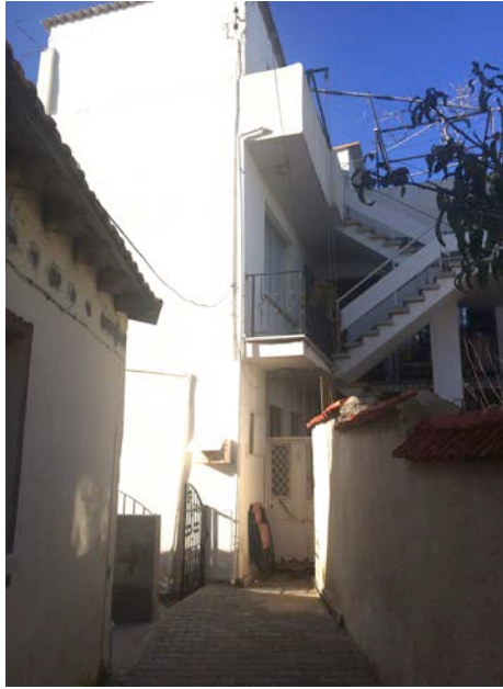
Figure 41: One and two storey attached buildings in ST5
