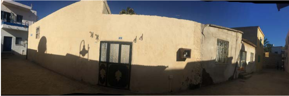
Figure 19: View of adjacent buildings in Behran Pasha Street
