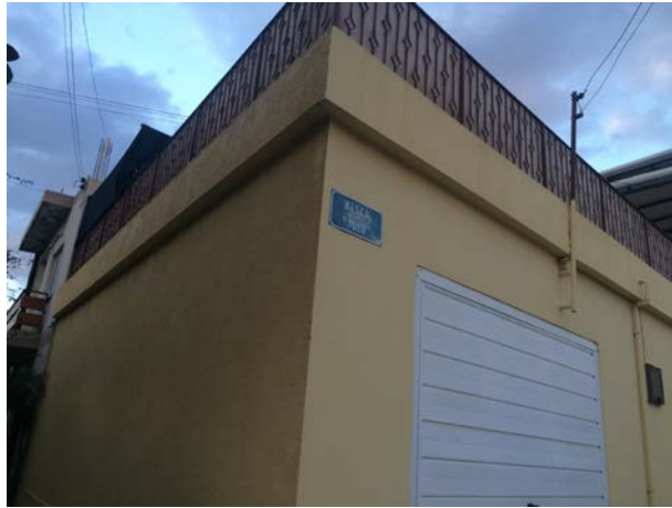
Figure 62: View of terrace in Kışla Yolu Street
