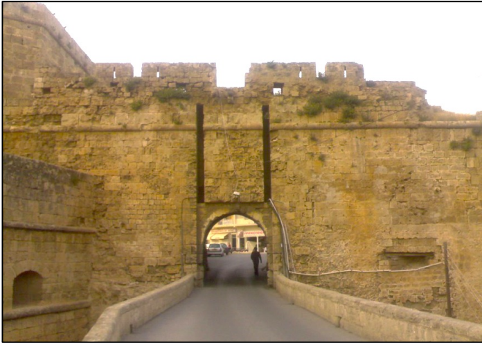
Figure 4.25: Akkule gate (Land gate), main entrance to district 2 and 3
