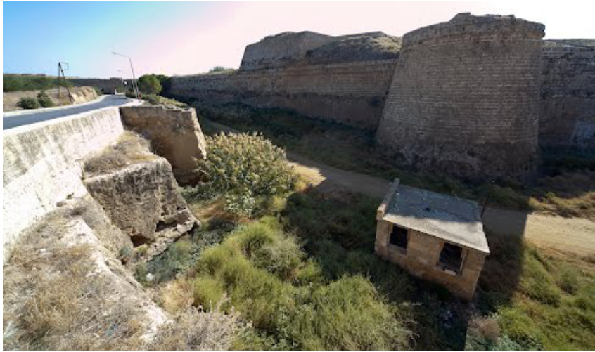
Figure 4.14: District 8, walls, ditch and towers
