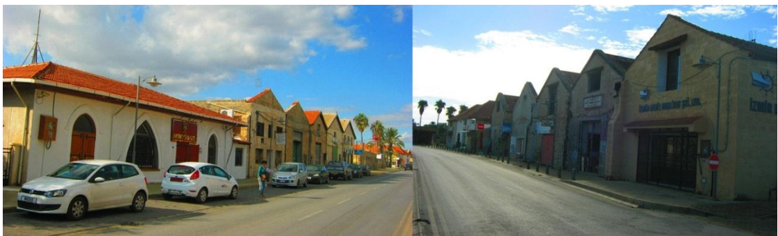
Figure 26: Warehouses along the Canbulat Avenue (Taken by author, 2013)
