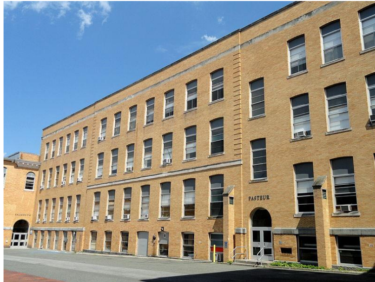
Figure 10: University of Lowell in a rehabilitated mill complex
