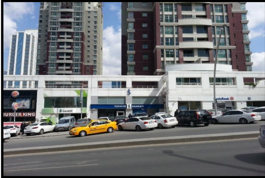
Figure 60: Ground level façade, Hayat Sebla Evleri
