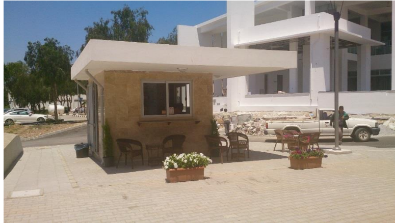
Figure 5.11: Public open spaces around accounting office
