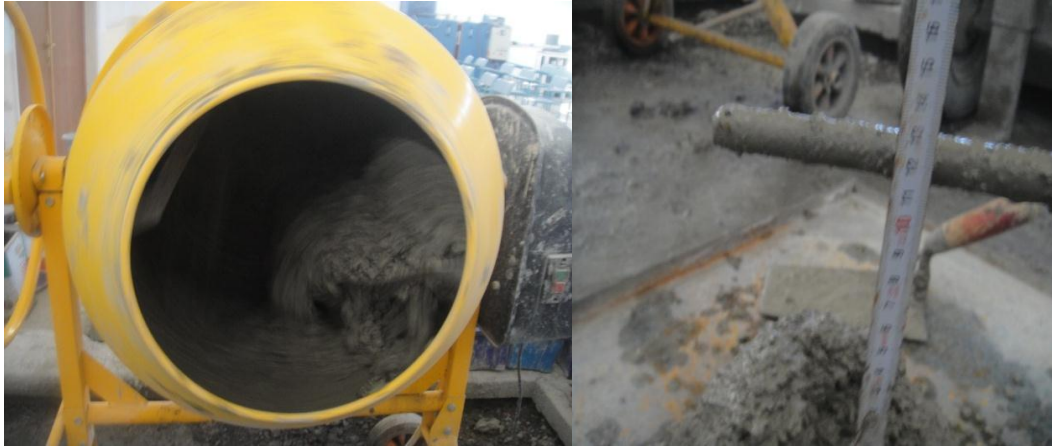
Figure 3.1. Mixing and slump test of fresh concrete
