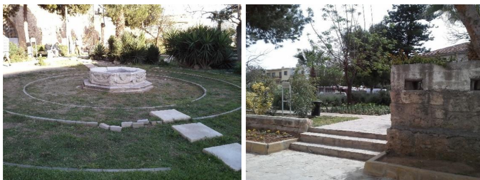
(a) Poor design of the landscape; grass condition (b) Entrances condition, the first impression
