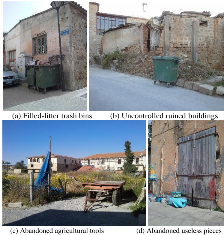
Figure 4.14: Existing condition of streets' maintenance in the Walled City, by author
