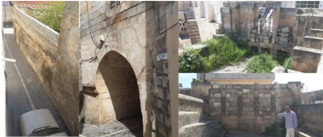
Figure 116: Views of Hac Recep Isgurgu Kabaltı house
