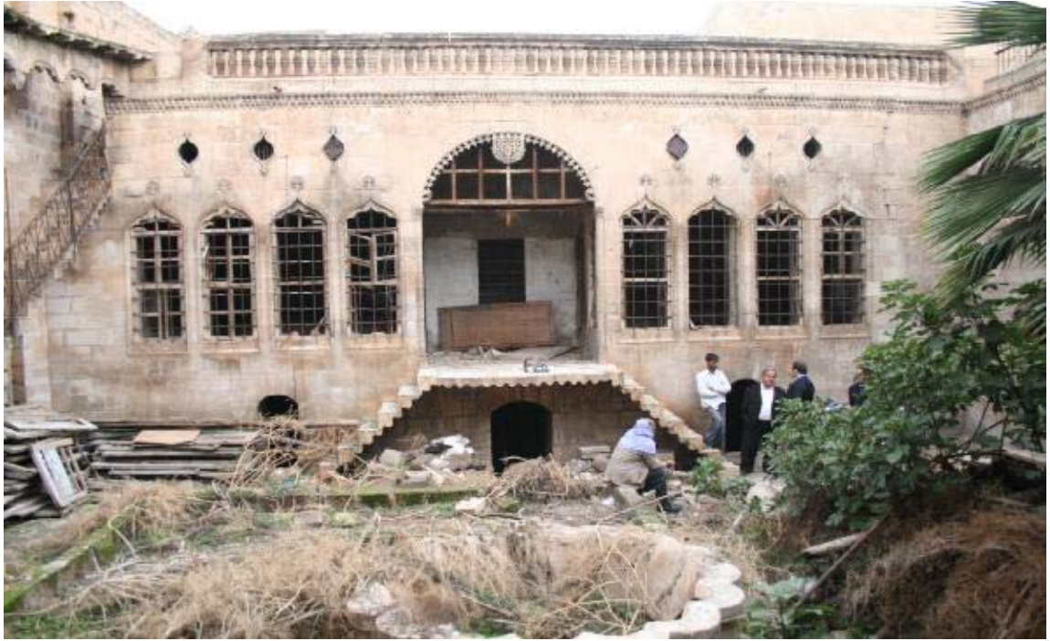
Figure 73: The reflection of the eyvan onto the internal façade, Akyüzler house, Urfa
