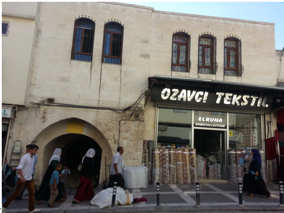
Figure 125: View of Salih Avcı Kabaltı House
