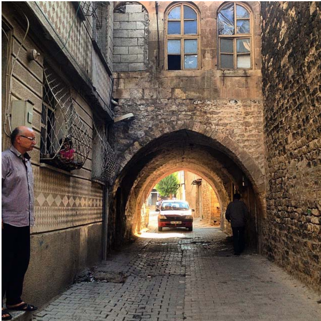
Figure 57: Utilization of kabalti space does not hinder and damage the public right of the way. (The Kabalti house in Kilis in Turkey)
