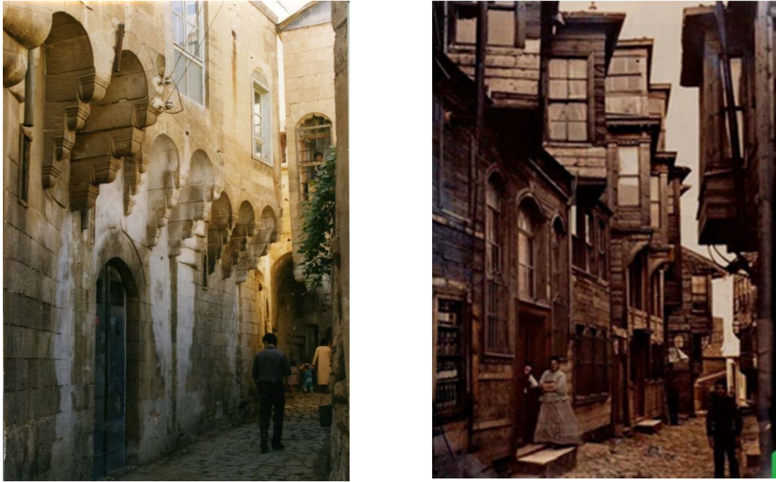
Figure 19: Façade articulation as projection in traditional settlement Anatolia (Source: Cahit Kürkcüoğlu Archive)
