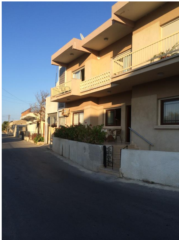
Figure 19. Good Structural Condition, (Street 2) Source: (Davoodi, 2014)
