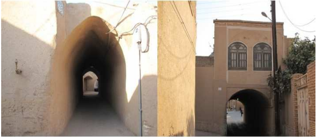
Figure 28: Roofed alleys in Fahadan area, Yazd/Iran
