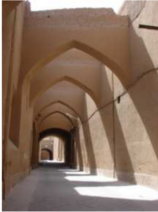
Figure 35: Structural role of roofed alley as beam
