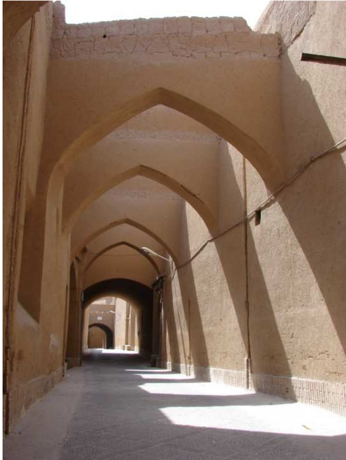
Figure 7: Combination of sun light and shadow by roofed alley
