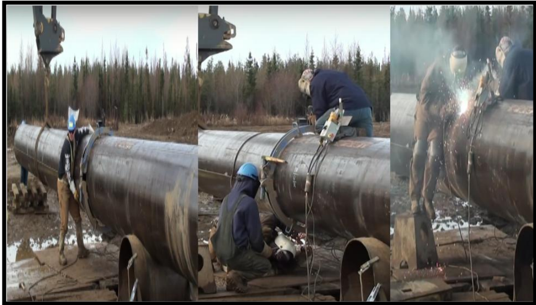
Figure 3.2: The Process of the Pipeline Installment on the Shore
