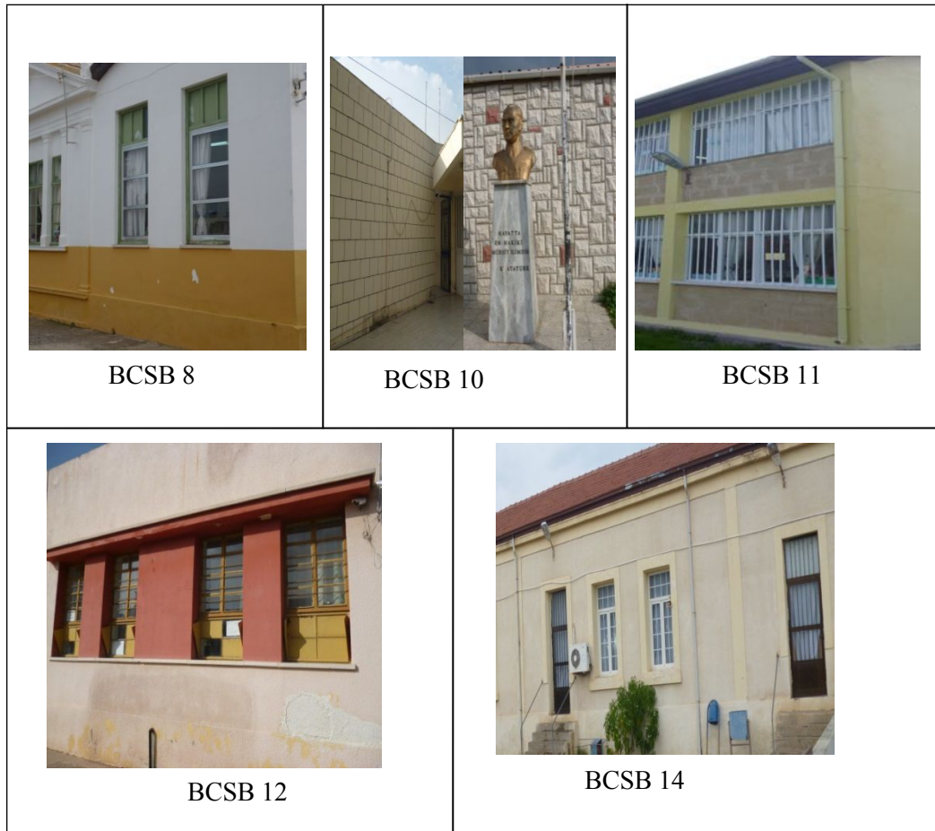
Figure 87: Wall structural systems from Famagusta cases (BCSB 8-Gazi ilkokulu , 10-Polatpasa ilkokulu 11-Canbulat ilkokulu, 12-Alasya ilkokulu and 14-Sehit Huseyin Akil ilkokulu)
