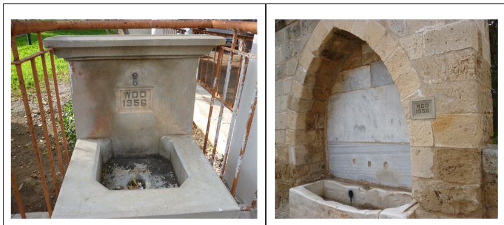
Figure 33: Concrete water supply channels in British period
