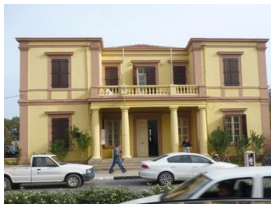
Figure 31: Gazimagusa Post Office
