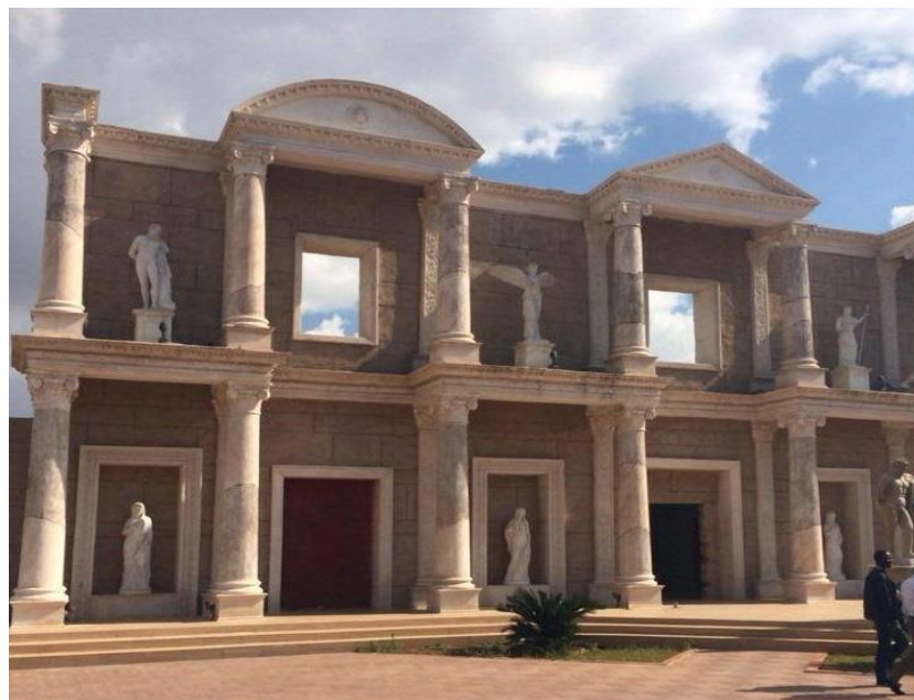
Figure 62. Kaya Artemis Resort exterior (Author, 2015)
