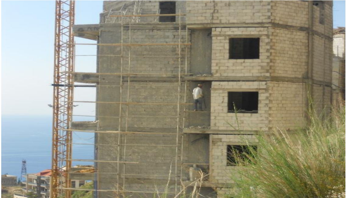
Figure 7. Old scaffold supporting system.
