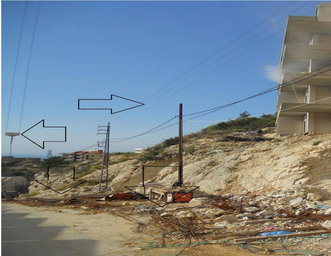
Figure 10. Lifting reinforcing steel bars using a tower crane near electric pole.
