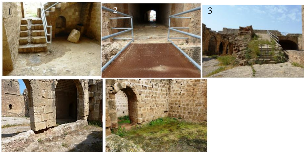
Figure 3.39: Different parts of intermediate level of Ravelin Bastion, (UNDP-PFF, Ravelin Bastion project, 2016).
