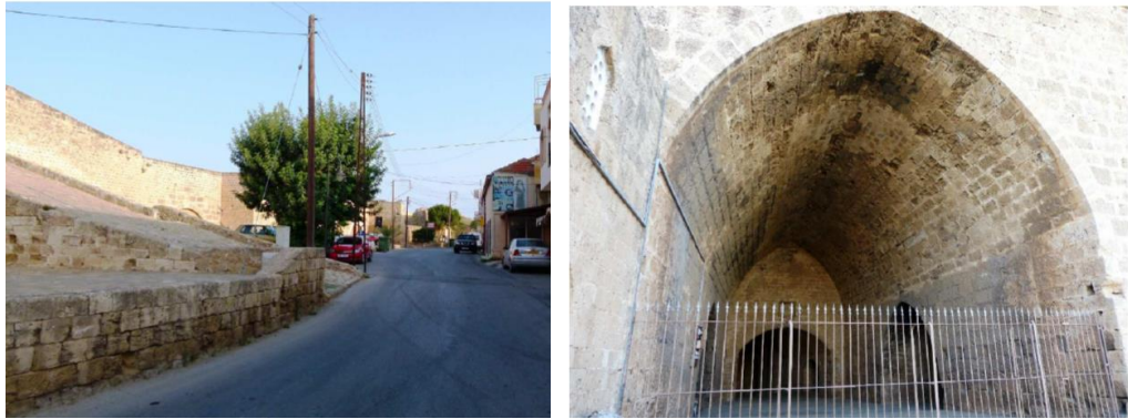
Figure 3.31: Main access and entrance to Ravelin Bastion (UNDP-PFF, 2016).
