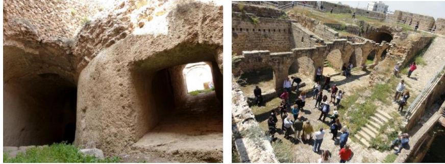
Figure 3.42: Tunnels and rooms inside Ravelin Bastion, photo from (UNDP, 2016)
