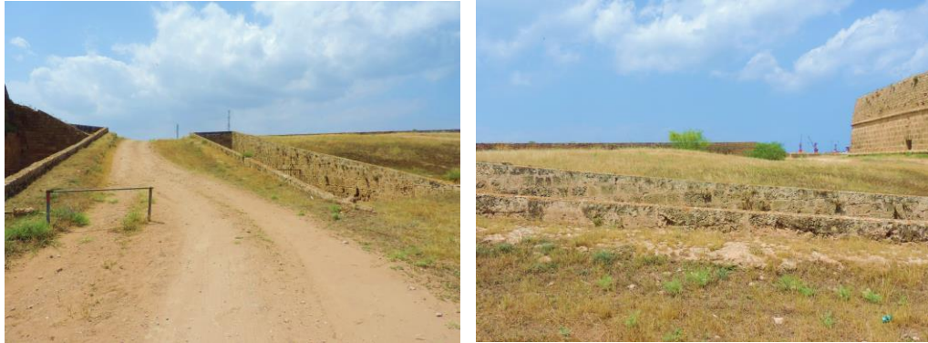
Figure 3.23: Access to roof of Martinengo Bastion through two ramps, (Author, 2016).
