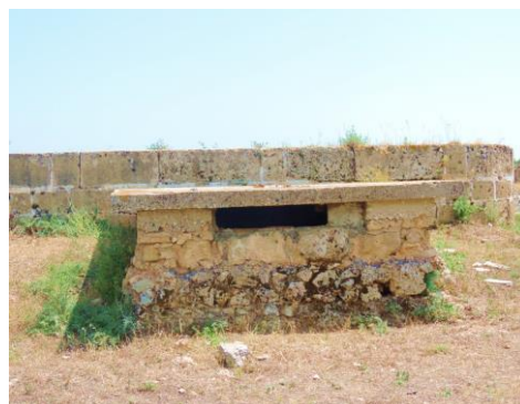
Figure 3.24: Chimneys for gunpowder smoke on the roof, (Author, 2016).
