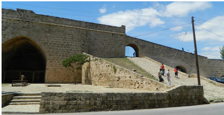
Figure 3.32: Access directly from road, (UNDP-PFF, 2016)
