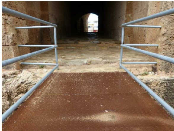
Figure 3.33: Metal bridge that has been replaced with drawbridge (UNDP-PFF, 2016)
