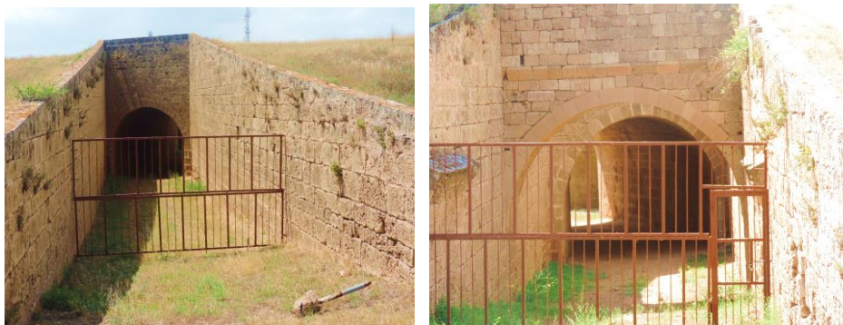
Figure 3.22: Sloping entrances into inside of Martinengo Bastion (Author, 2016).
