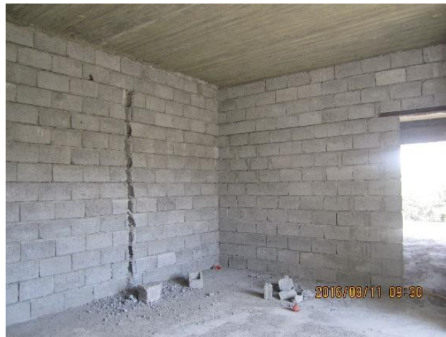
Figure 23: Lack of Thermal Insulation for the Roof (Taken by author, 2016)
