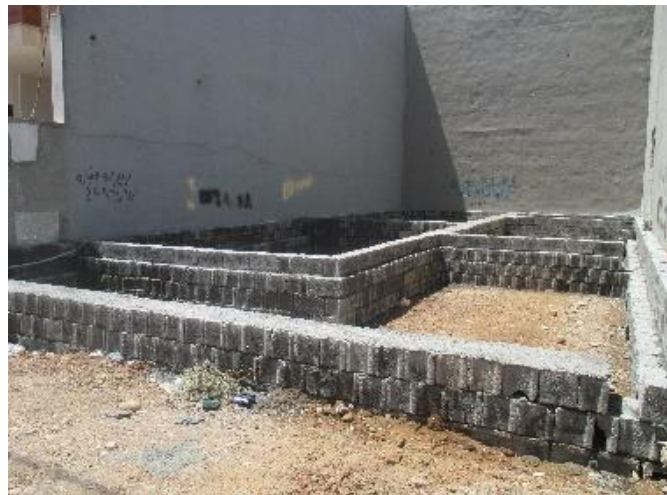
Figure 15: Construction of Foundation Via Block Work (Taken by author, 2016)
