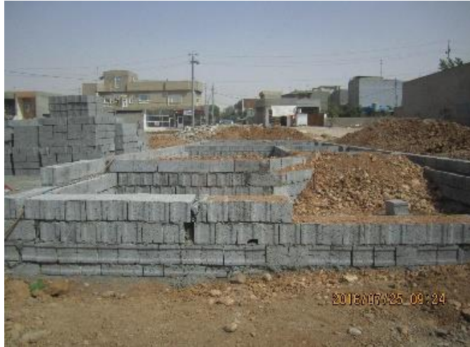
Figure 14: Settlement and Soil Test for Land (Taken by author, 2016)
