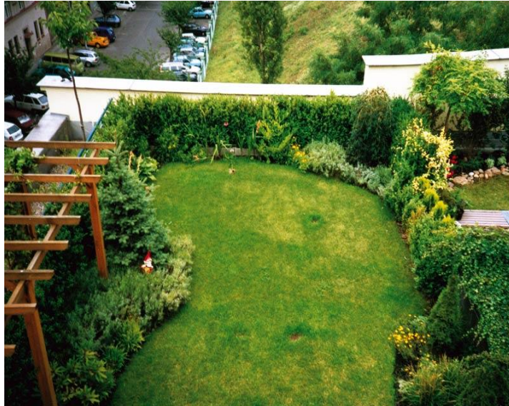
Figure 2: Intensive Green Roof [4]
