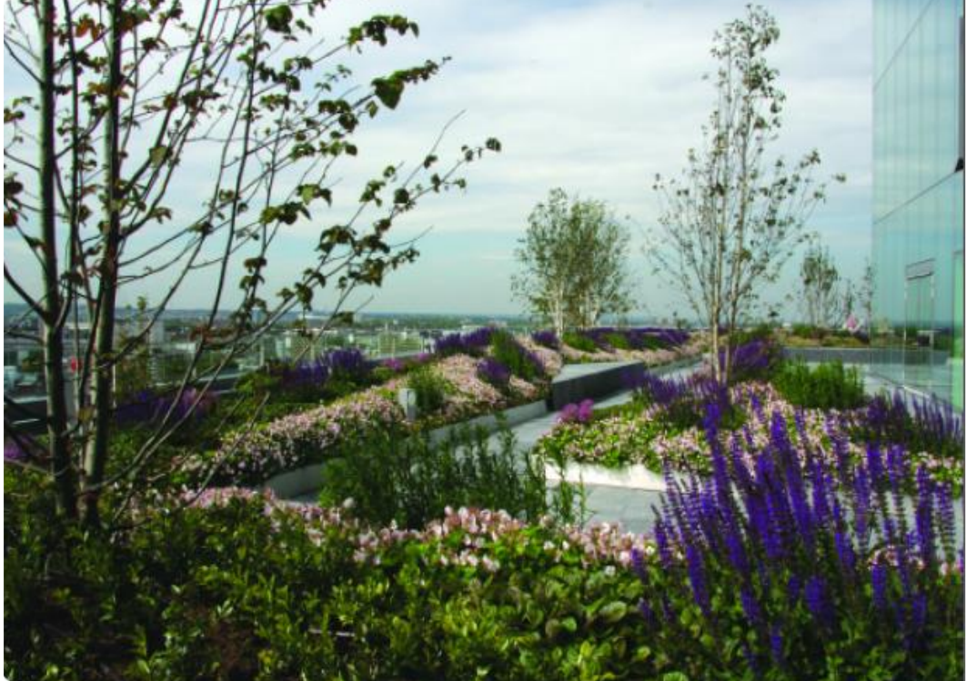
Figure 4: Accessible green roof on a new office development, Islington [5]
