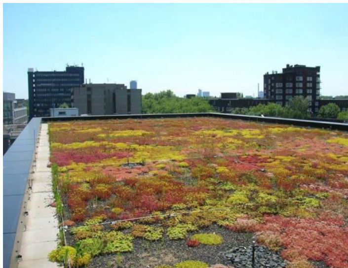
Figure 1: Extensive Green Roof [3]
