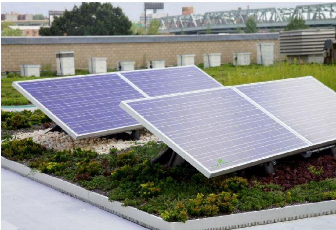
Figure 4.10: Green Roof with solar panels [50]
