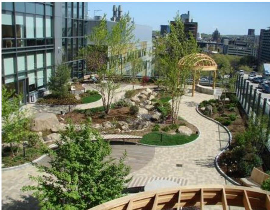
Figure 2.3: Intensive Green Roof [6]
