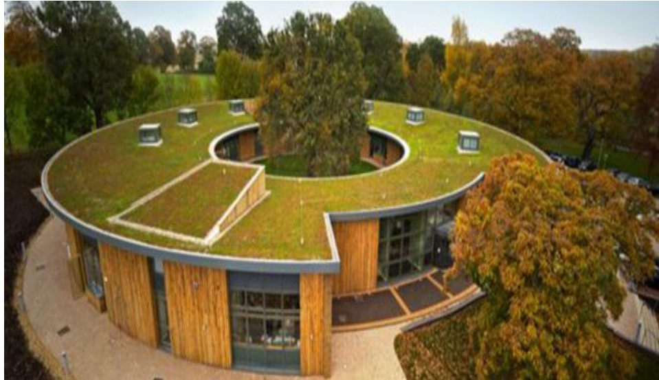
Figure 2.2: Extensive Green Roof [5]
