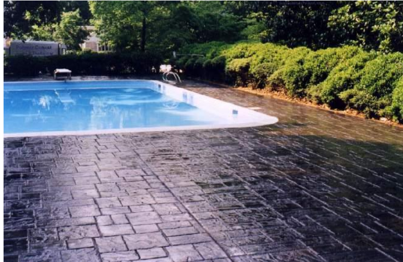
Figure 2.15: Application of Polymer Concrete [22]
