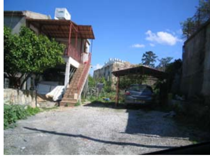
Garage located on aside of the house
