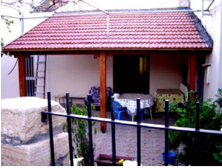
Semi-open space addition in front of the main entrance
