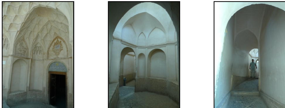
Figure 2.6. Entrance, Hashti and Dalan (left to right) in a traditional Iranian house
