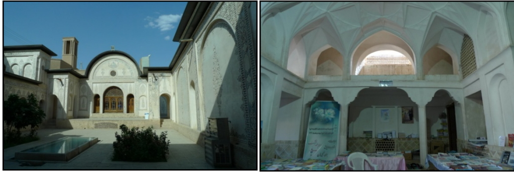
Figure 4.12. View from outside and inside of the basement in a traditional Kashani house
