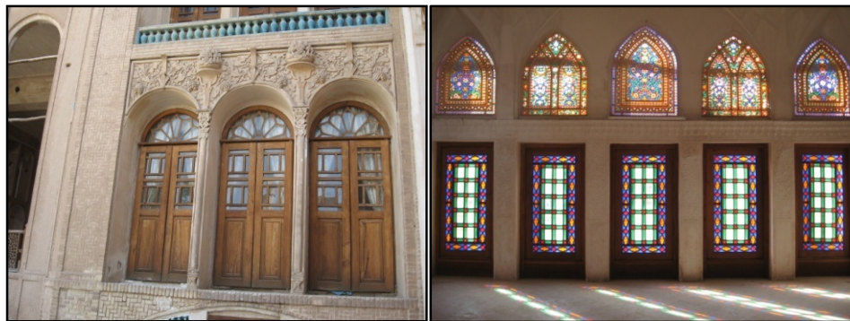
Figure 2.9. A Seh-dari (left) and a Panj-dari (right) in a Traditional Iranian House
