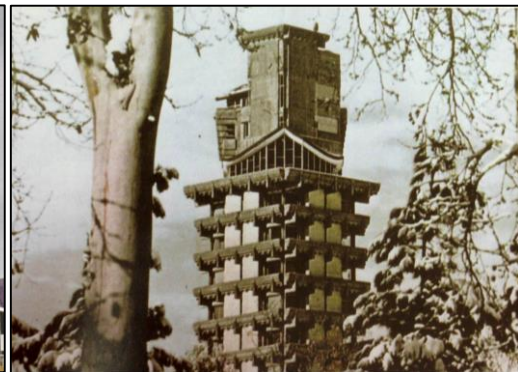
Figure 53: Construction with exposed concrete in Structuralism style by Jahangir Darvish during 50's, (Bavar, 2008, p. 144)
