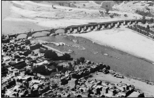
Figure 45: Example of ne transportation facilities, Dezfoul Old Bridge, (Bavar, 2008, p. 52)
