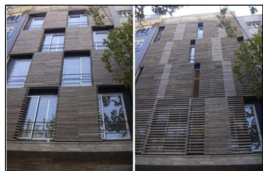
Figure 81: Flexible, dynamic surface of the façade in Khorana Office Building by Rambod Eilkhani, (Eilkhani, 2012)
