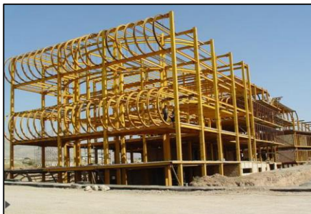
Figure 63: Steel structure in Asr Danesh Afzar Building by Arash Mozaffari, (Mozaffari, 2005)
