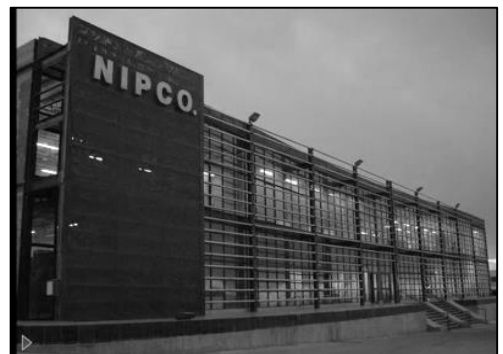
Figure 77: Idea of an opaque center covered with a transparent shell in NIP Co. by Arash Mozaffari, (Mozaffari, 2005)
