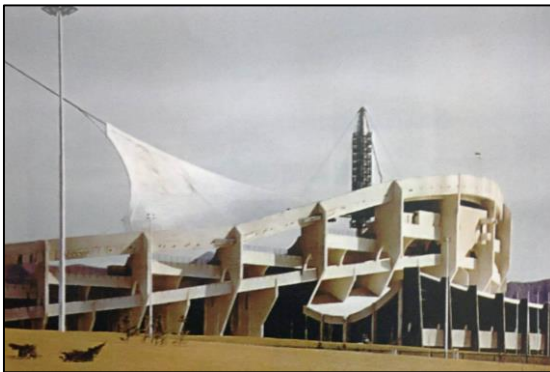
Figure 52: Takhti Stadium with tensile cable structure during 1970 by Jahangir Dervish, (Bavar, 2008, p. 141)
