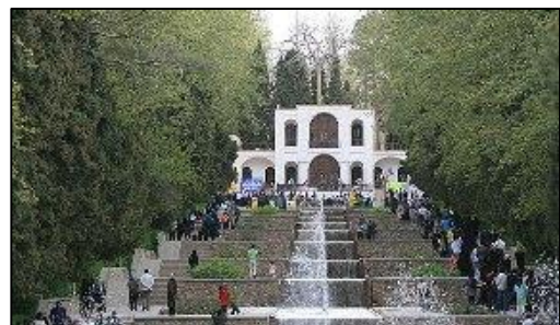
Figure 76: The central building in Shazdeh Garden, (Bultannews, 2011)
