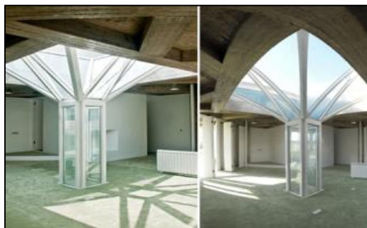
Figure 132: Play of light through interior spaces in Dervish Villa by Pouya Khazaeli, (Khazaeli, 2010)
