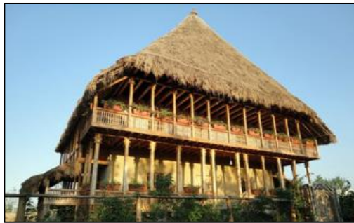
Figure 97: Traditional houses with gable roof in humid areas, (Abela & Aguilar , 2007)
