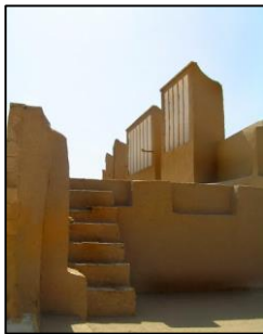
Figure 109: Usage of roof in traditional houses, (Fotoohi, 2009)
