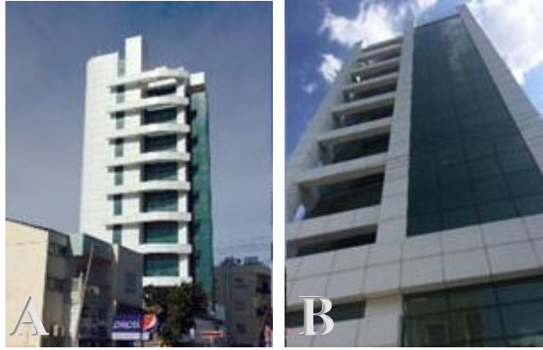
Figure 3.22. Shading Devices and Glazing on the UMK's North and South façades
