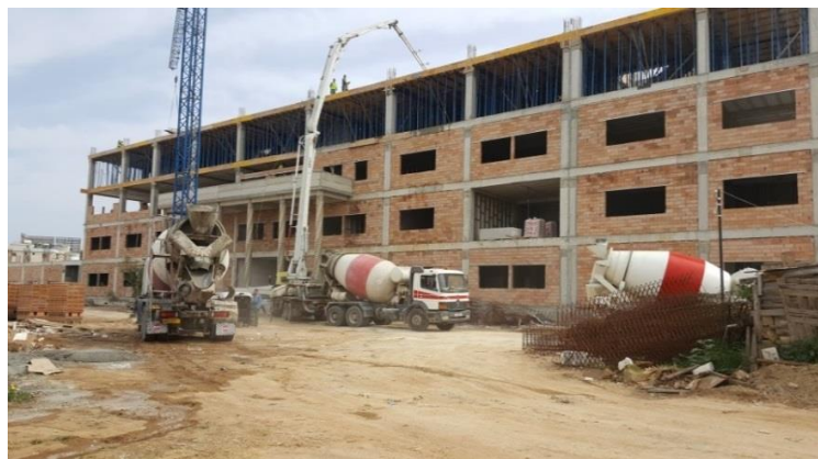
Figure 20: Construction Jobsite View
