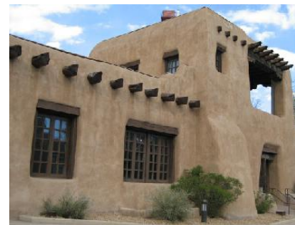
Figure 4.18: Timber roof and slab in adobe masonry building (URL 5)
