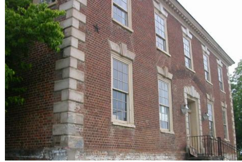
Figure 4.15: Examples of stone and brick building which have interlocked corners (by author)
