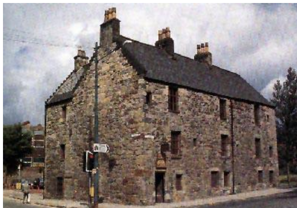
Figure 4.22: Traditional stone building (by author)
