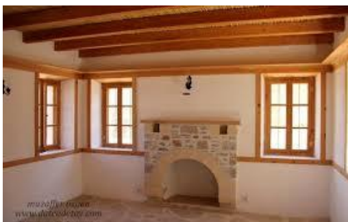
Figure 4.17: Timber roof and slab in masonry building (Kucukerman, 1991)
