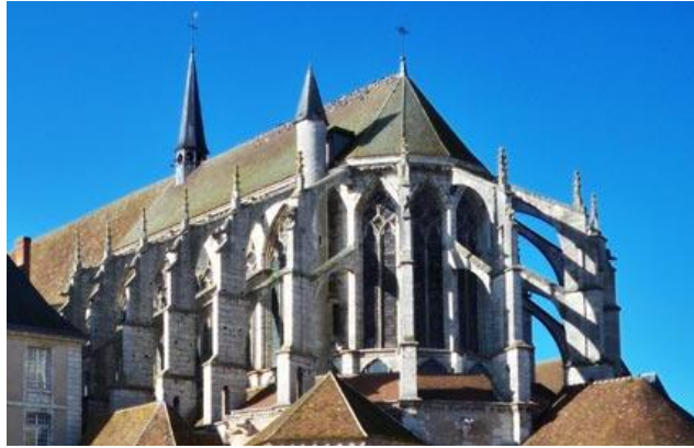
Figure 4.21: Flying buttresses of the Gothic Architecture (URL 4)
