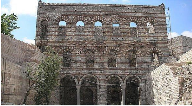
Figure 4.12: Brick and stone layers on wall (Tekfur Palace) (URL 4)
