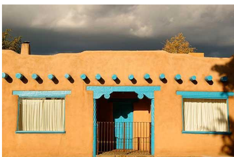
Figure 4.18: Timber roof and slab in adobe masonry building (URL 5)
