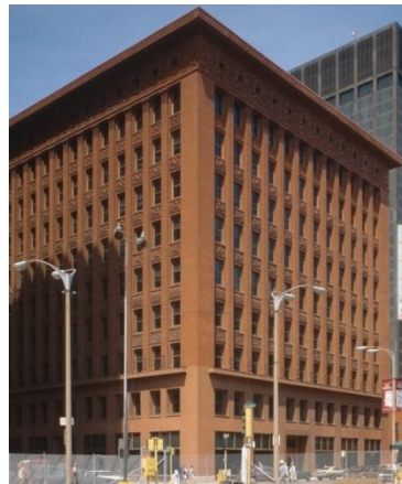
Wainwright Building (1890), by L. Sullivan (Rolf, 2013)
