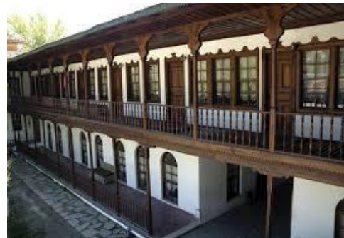
Figure 4.17: Timber roof and slab in masonry building (Kucukerman, 1991)
