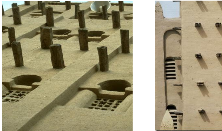
Figure 4.33: Horizontal timber elements, repeated openings and buttresses on adobe wall (URL 5)
