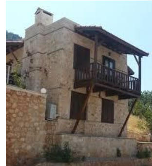
Figure 4.13: Stone masonry with timber horizontal ties (by Author)
