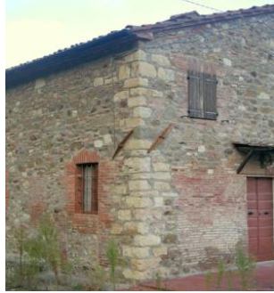
Figure 4.15: Examples of stone and brick building which have interlocked corners (by author)
