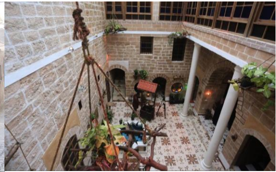
Figure 54: Restored Salama House with Same Residential Function (Source: Iwan Centre, 2016)
