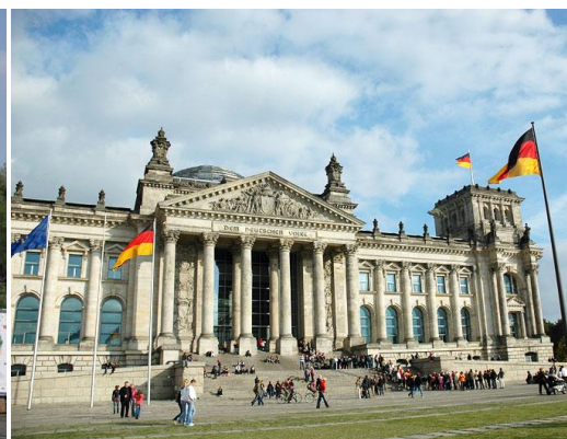
Figure 15: Historical Building in Berlin (Source: The German Way & More, 2016)
