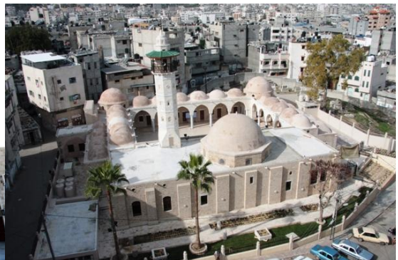
Figure 50: Restored Al-sayed Hashim Mosque (Source: Iwan Centre, 2015)
