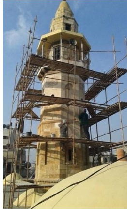
Figure 51: Conservation Works at Ibn Othman Mosque (Source: Iwan centre, 2016)
