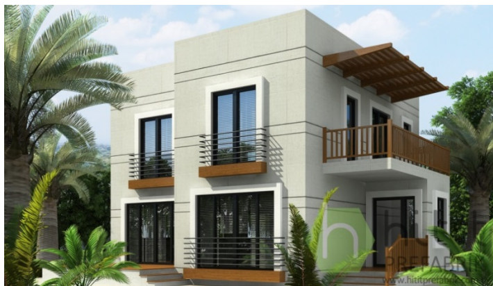
Figure 3.8. 'Steel construction homes' from the context 2 ©Hitit Prefabrik (URL 7)
