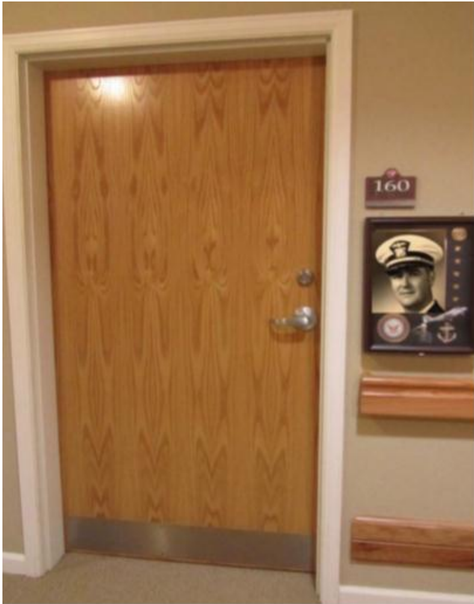
Figure 9: Locate Personal Photo and Memory Boxes Outside Each Bedrooms For Helping Way Finding (Marquardt, , 2009).
